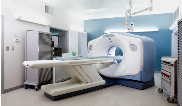
Figure 3. Supercapacitor UPS's are used in medical and healthcare environments primarily for bridge power, i.e. to bridge the gap when power is lost to when a generator starts up.
