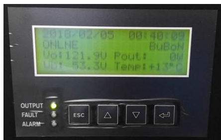
1. Fault LED on LED Shows a Fault
